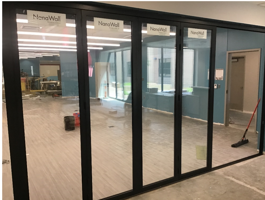
Folding glass partition installed.
