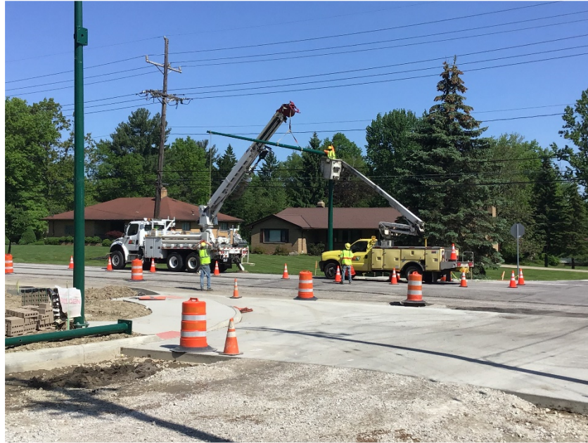
Installing traffic poles are Oaks Rd entrance.
