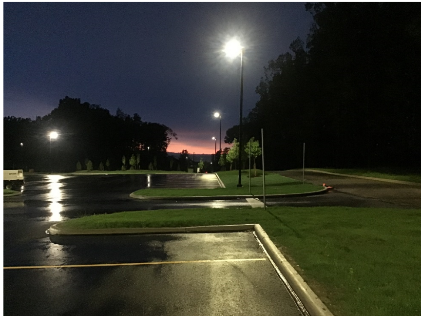
East parking lot asphalt, striping, and landscape complete.
