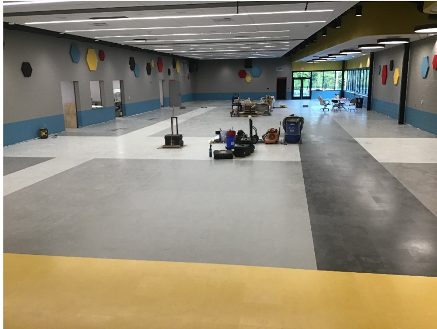
Flooring completed in Dining area.
