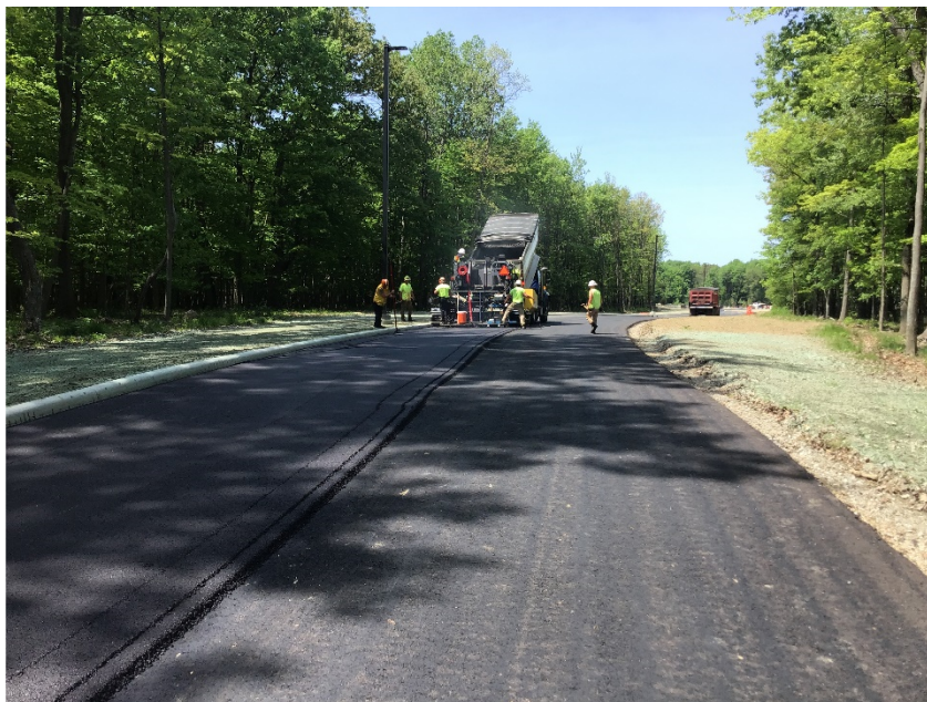
Laying surface course asphalt on drive to Valley Parkway.
