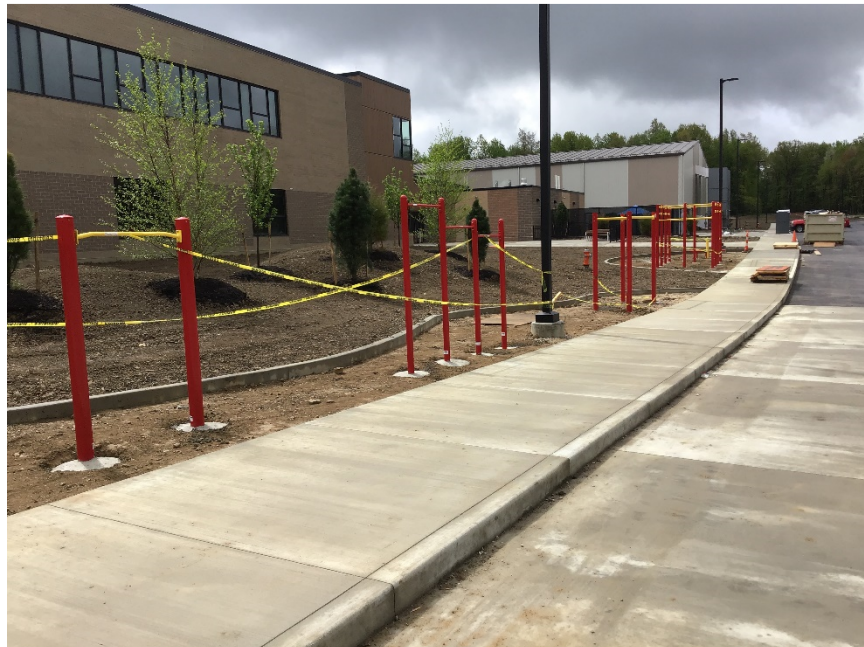
Playground equipment installation in progress.
