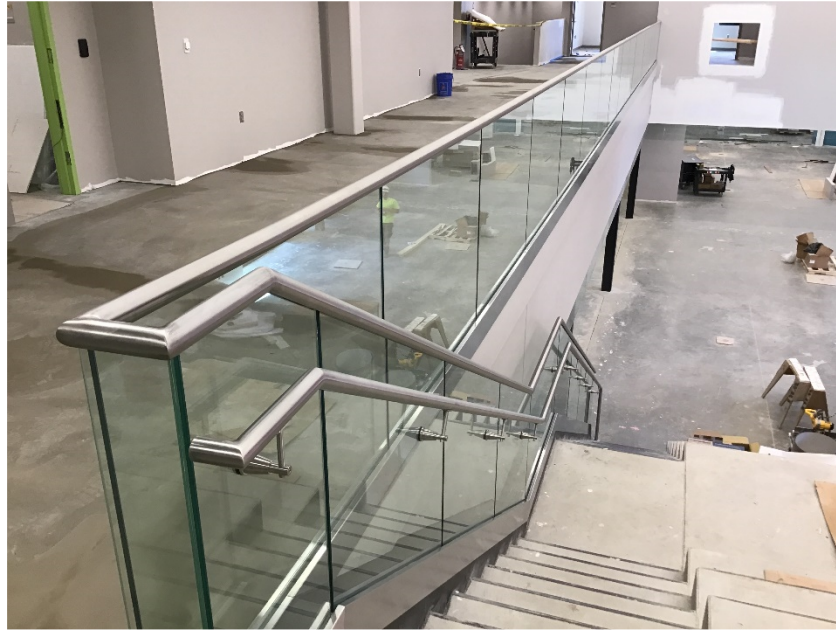
Glass handrail installed at Learning Stair.
