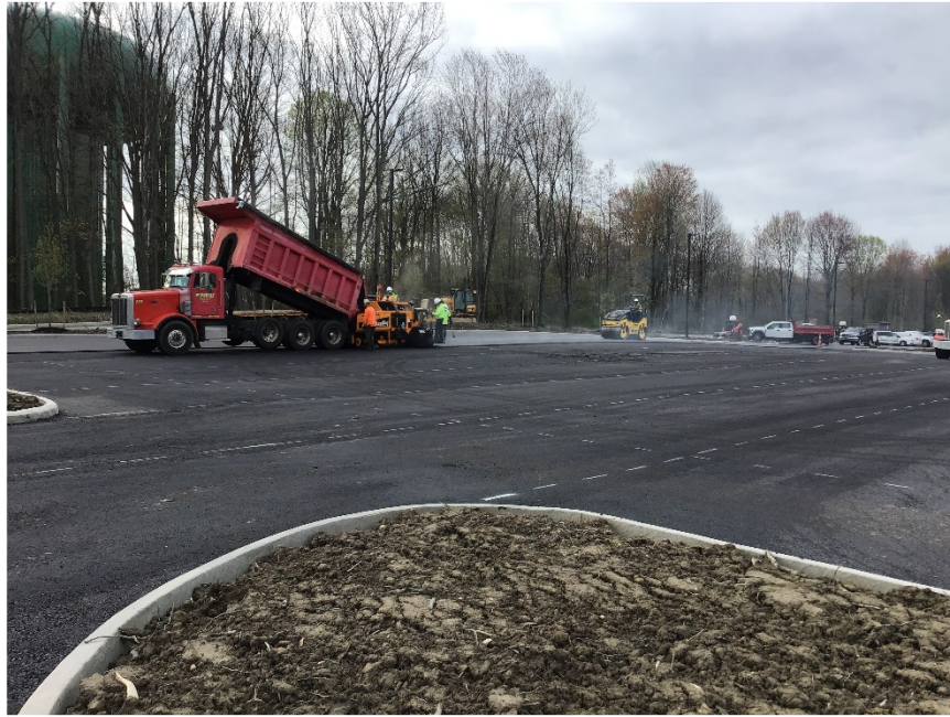
Paving surface course asphalt at East parking lot.
