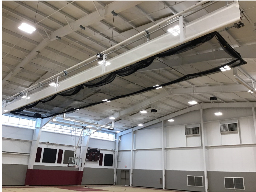
Batting cage installed.
