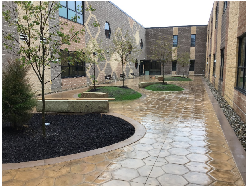
Courtyard landscaping complete.
