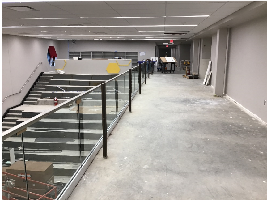
Glass handrail in progress at 2 nd floor / Media Center.
