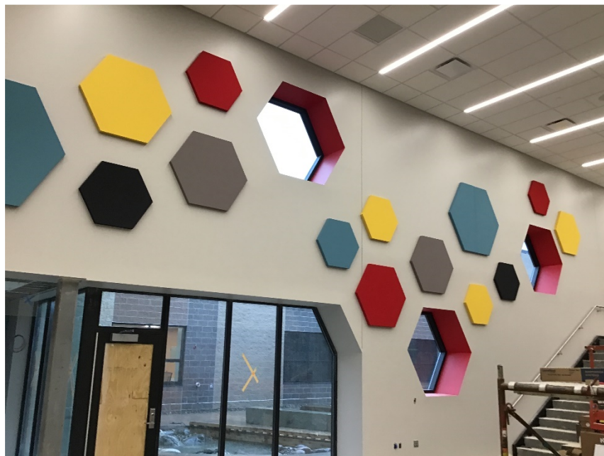
Acoustical panels installed in Media Center.
