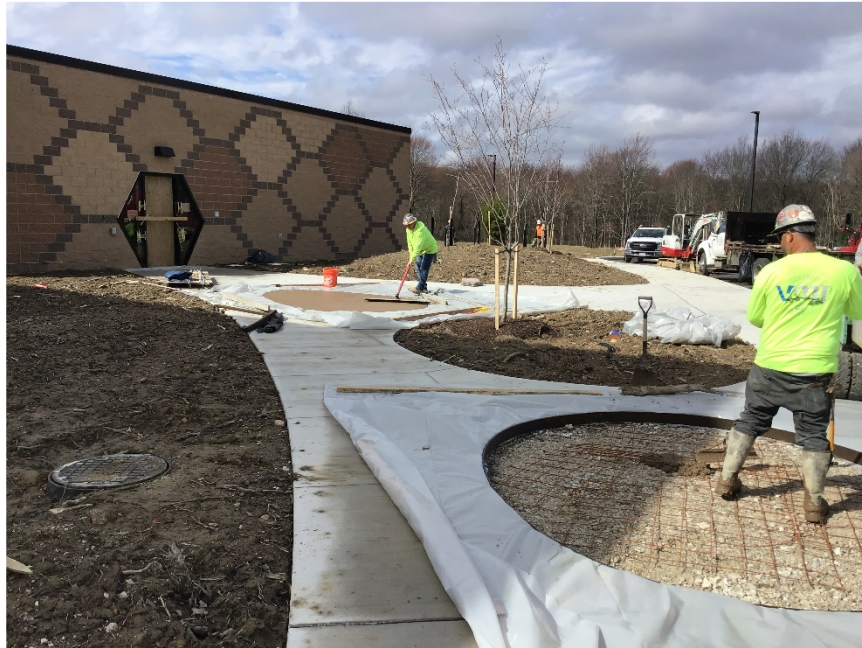
Pouring colored concrete infills at Pre-K drop off.
