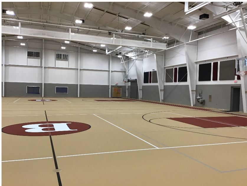
Fluid applied athletic flooring completed in Field House.
