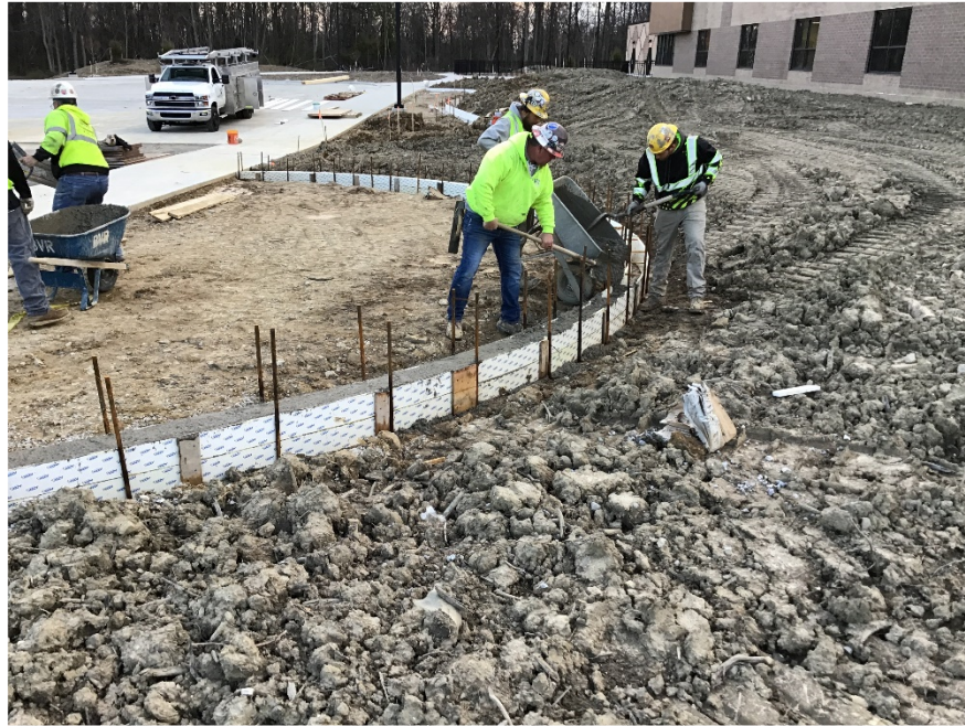
Pouring concrete curb for playground area.
