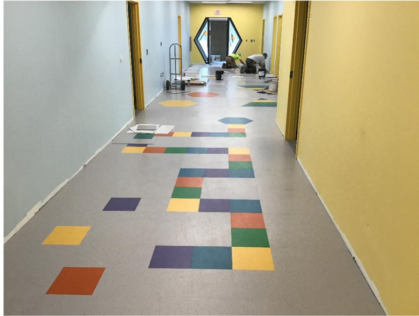
Flooring in Pre-K wing being installed.
