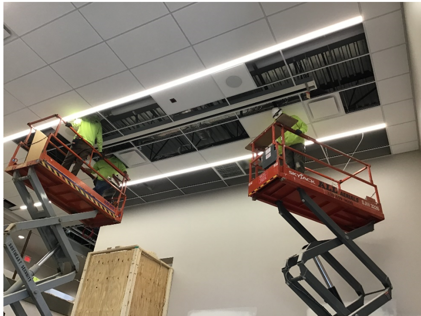
Installing ceiling pads in Media Center.
