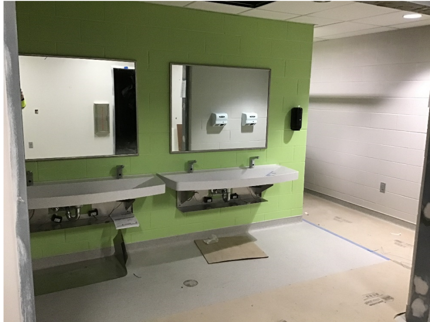
Plumbing fixtures in the process of being installed in Area 3 (2 nd / 3 rd Grade).
