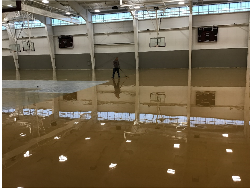
Fluid applied athletic flooring being installed in the Field House.
