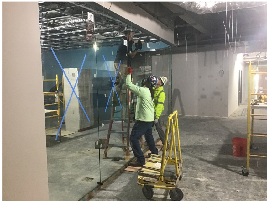
Installation of glass panels for the Makers Space.
