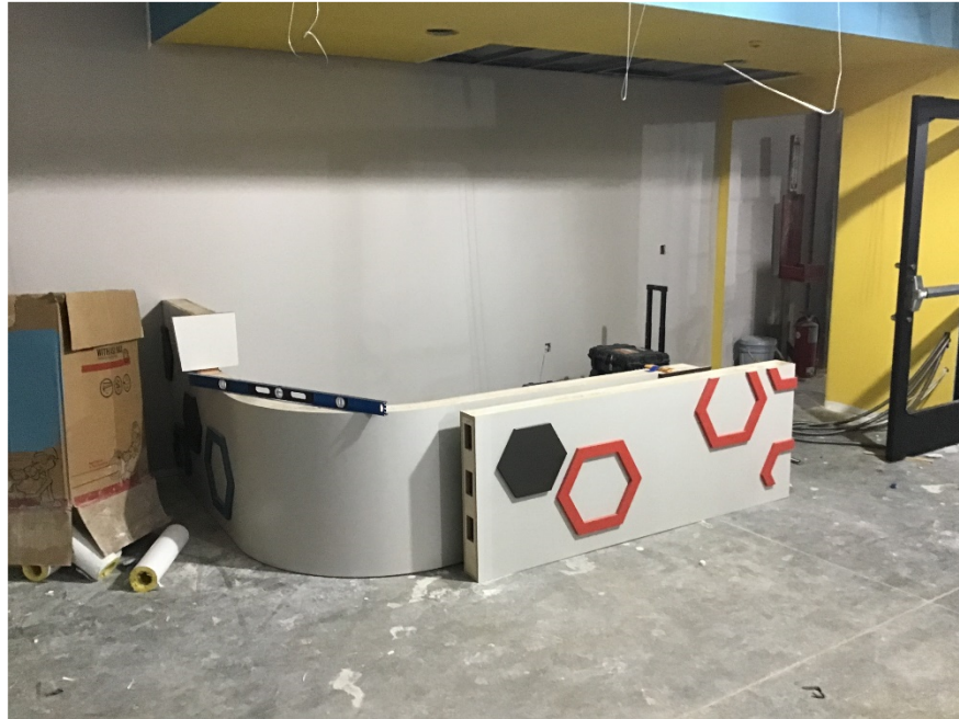
Casework in progress in Area 4.
