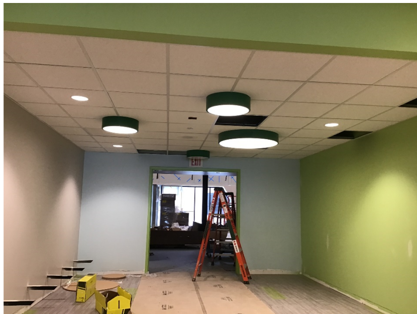
Light fixtures installed in the 2 nd / 3 rd grade wing.
