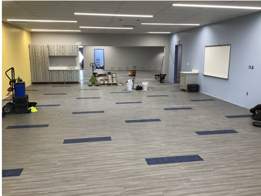
Finishes in progress in the 4 th / 5 th Grade wing.
