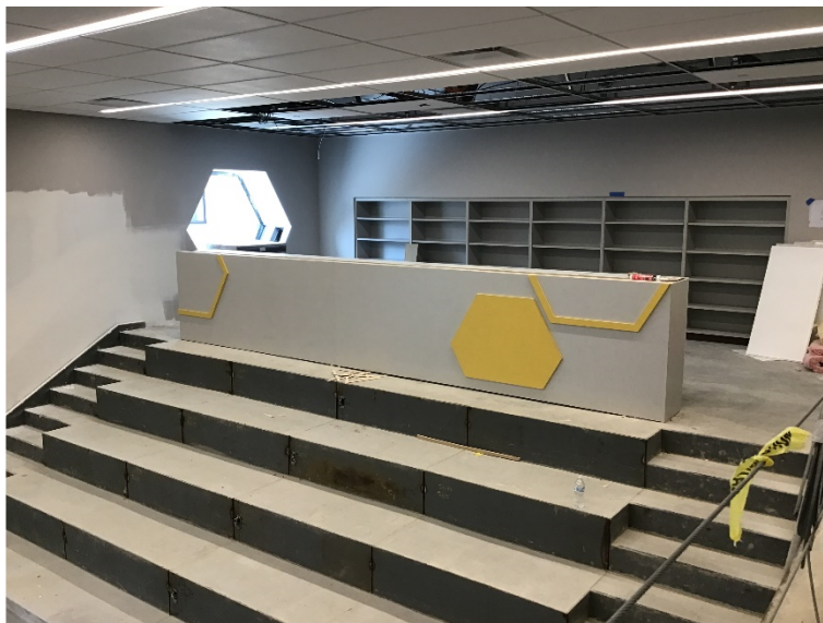
Casework at top of Learning Stair.
