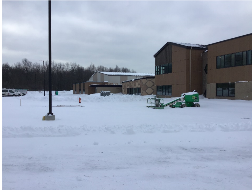
East elevation after February snow.
