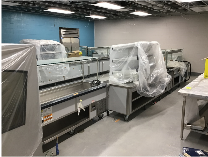
Kitchen equipment was delivered and set in place.
