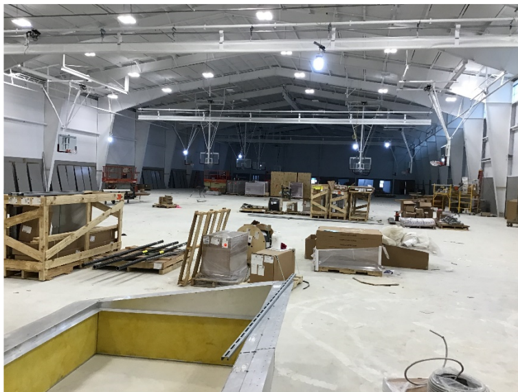
Field House backstops and curtains installed.
