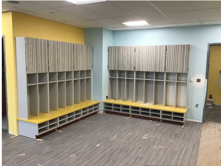
Classroom casework installation in progress in Pre-K.
