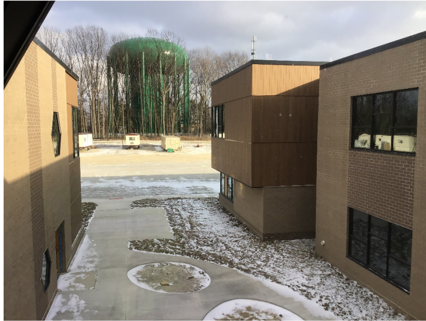
Alcove on the east elevation between Areas 1 and 3.
