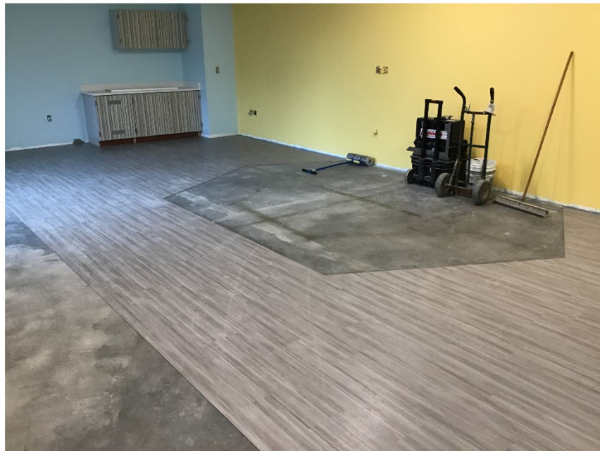
Pre-K flooring in process of being installed.
