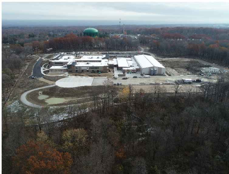
Arial view looking East.
