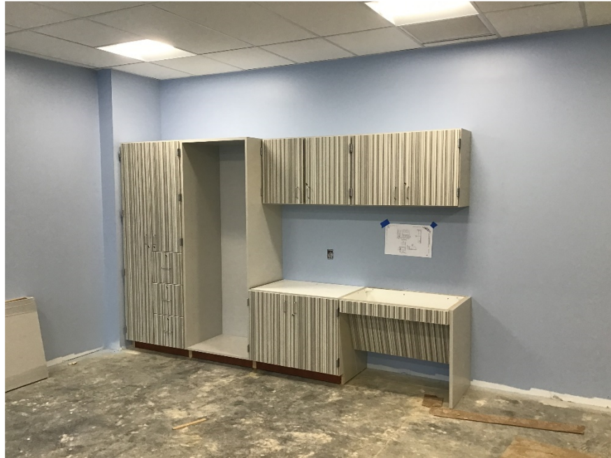
Classroom casework installation in progress.
