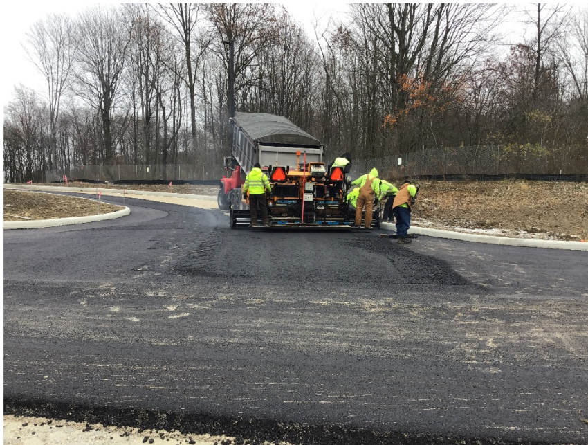
Installing base course asphalt for Pre-K drop of lane.
