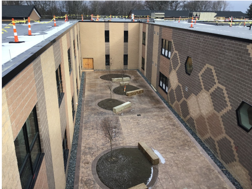
Stone benches and landscaping installed in Courtyard.
