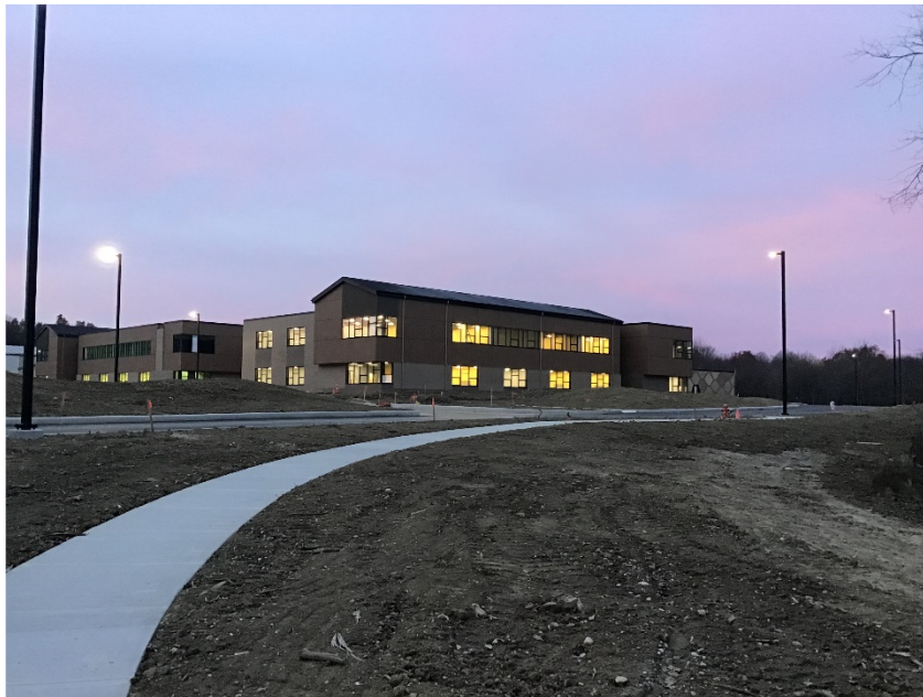
North elevation / 4 th and 5 th grade wing.
