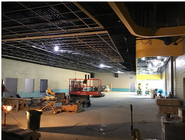
In progress of installing acoustical ceilings in the Student Dining area.
