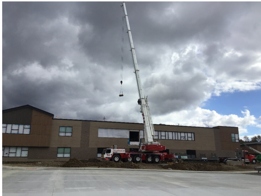
Crane setting stone benches in Courtyard.
