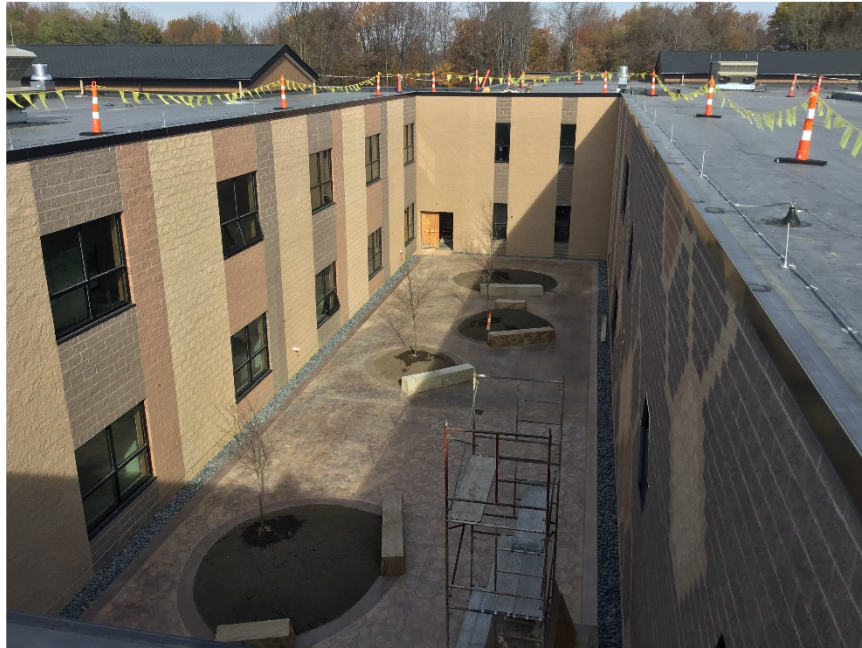
Stone benches and landscaping installed in Courtyard.
