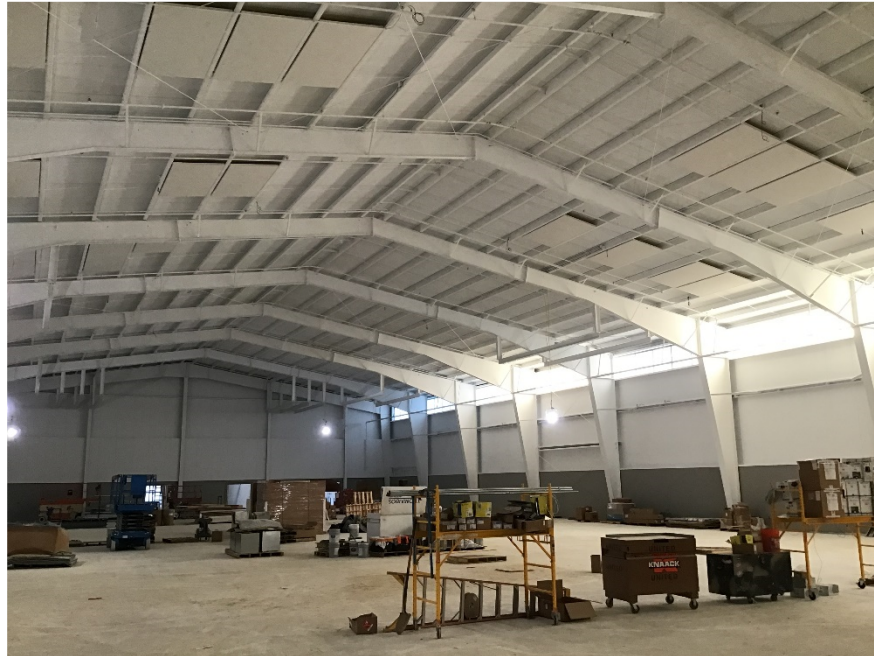
Acoustical panels being installed in Blossom Field House.
