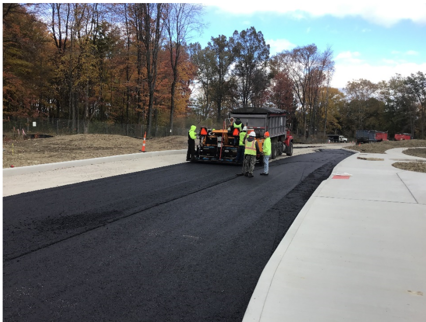
Laying base course asphalt on north side of building for Pre-K turn around.
