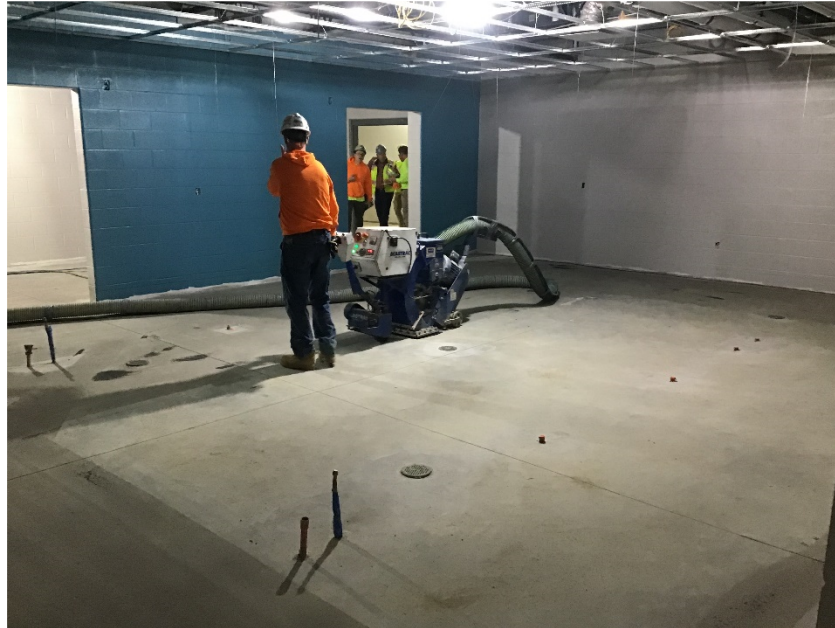
Grinding floors in kitchen in preparation for resinous flooring.
