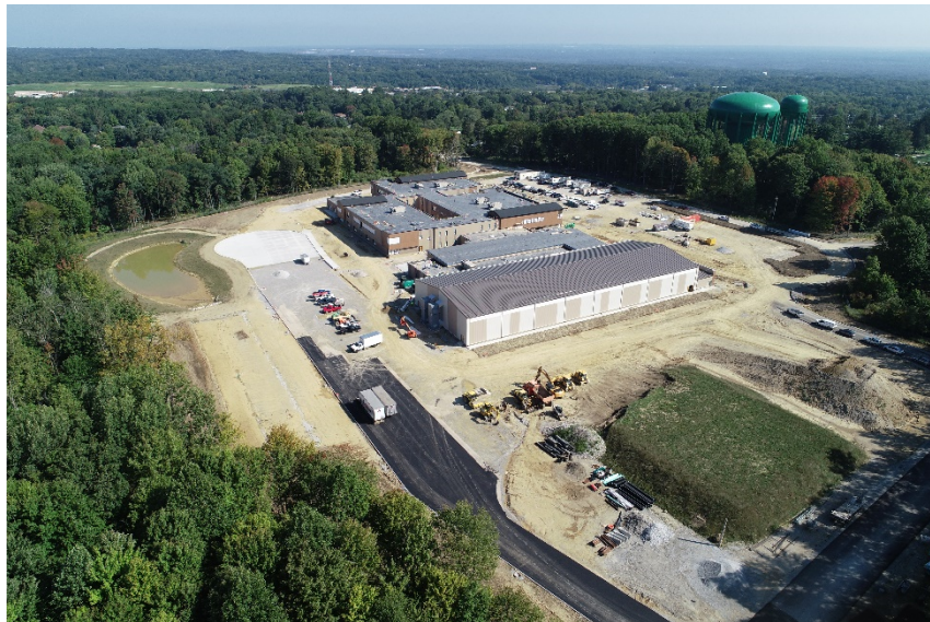
Overall view looking northeast.
