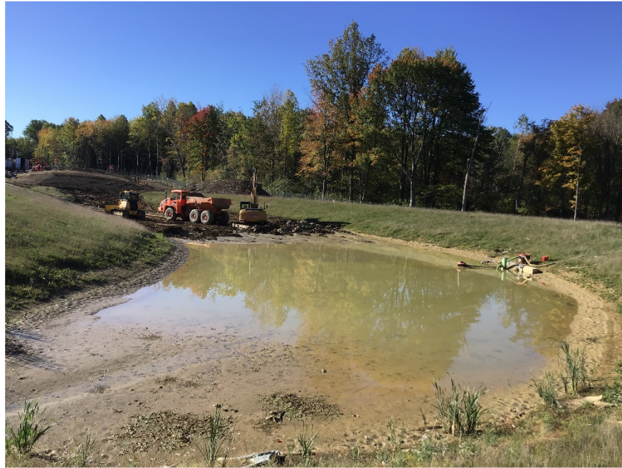
Regrading temporary sediment basin on West side of project.
