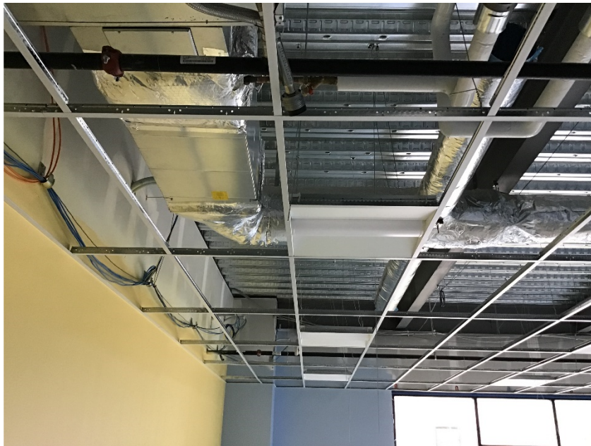
Acoustical ceilings and light fixtures being installed in Pre-K, 4 th , and 5 th grade wing.
