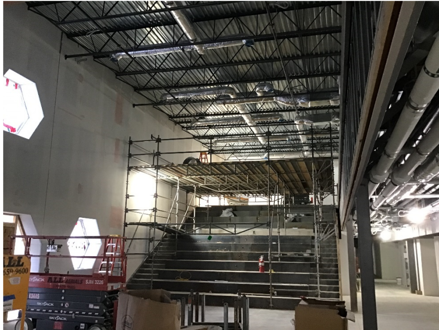
Temporary scaffold installed over the Learning Stair to allow overhead work to completed.
