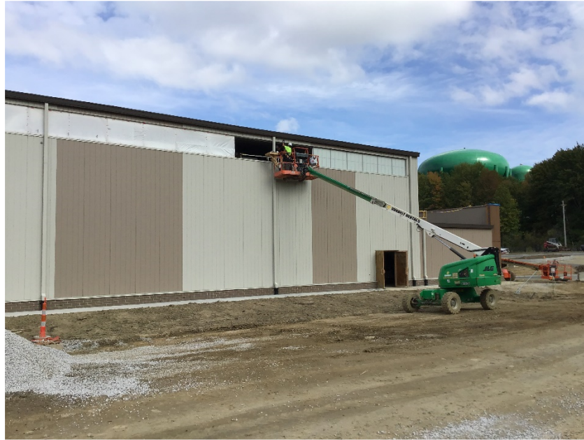
Installation of translucent panels on south elevation of Blossom Field House.
