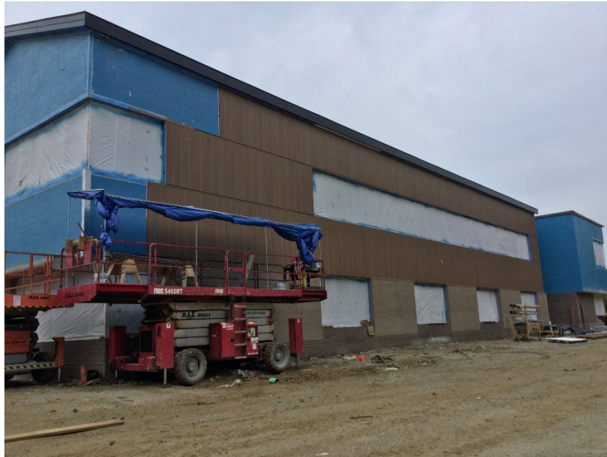
Fiber cement panel installation on East elevation.
