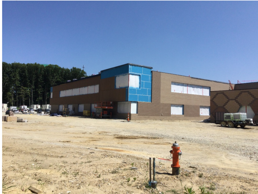
Overall view of north elevation.
