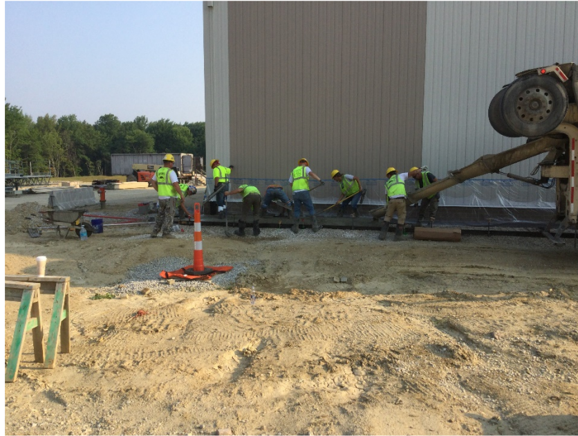
Concrete crews poured sidewalk on the south side of the Field House.
