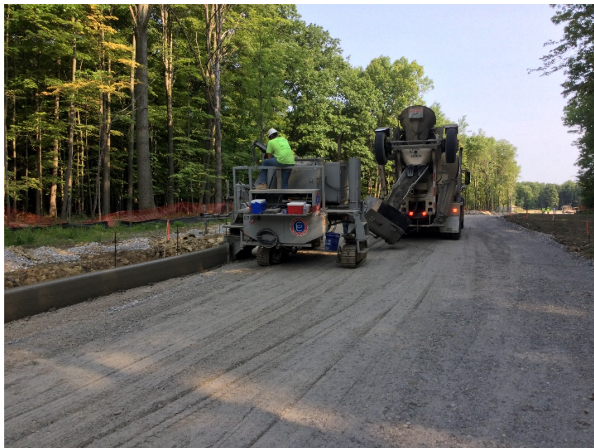
Concrete crews pouring curb on drive to Valley Parkway.
