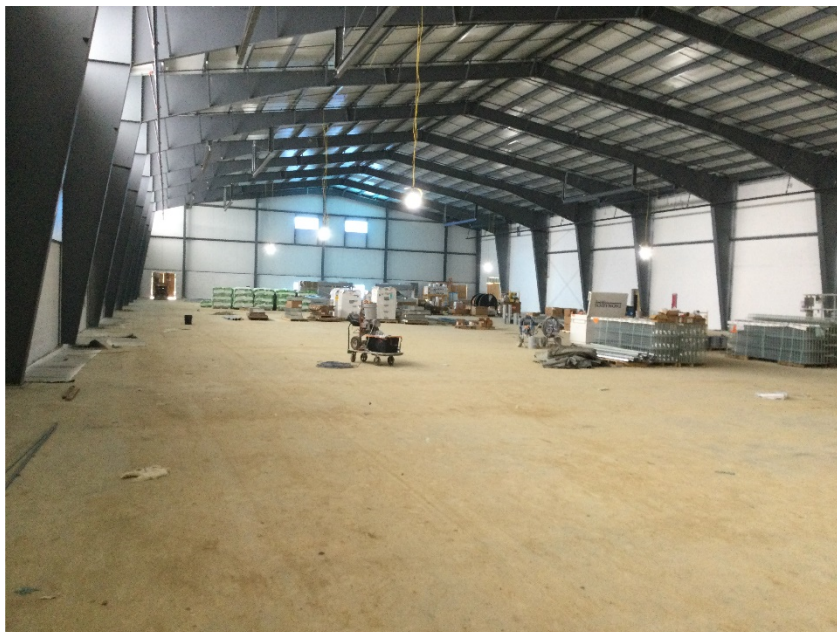
Field House overhead electrical rough in continuing.
