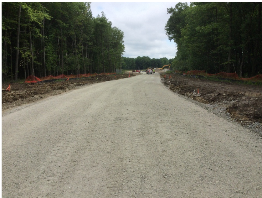
Stone base for road to Valley Parkway in progress.
