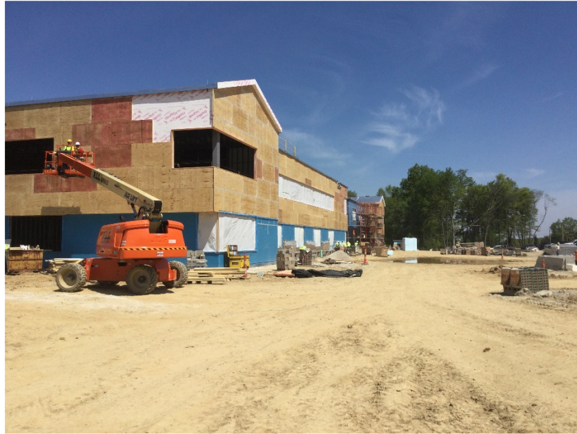
Hunter wall panel installation in progress 4 th /5 th grade wing.
