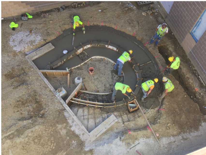
Pouring concrete for the Courtyard Pond.
