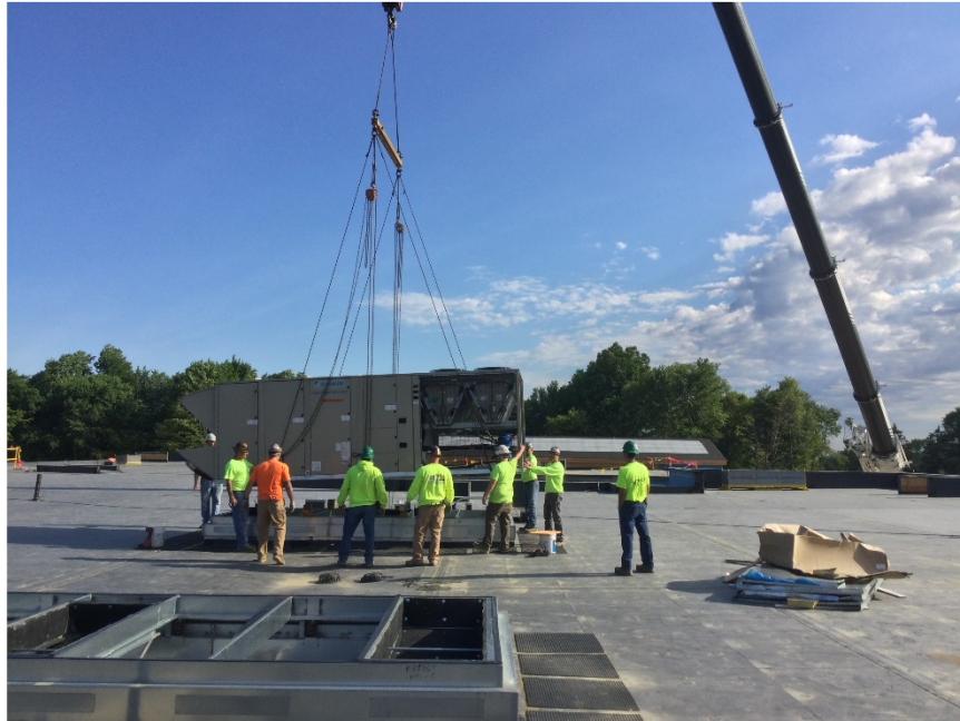
Setting mechanical roof top units.
