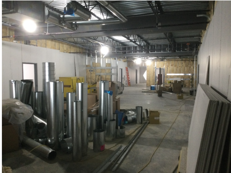
Drywall and insulation being installed in Area 1 (4 th /5 th grade wing).
