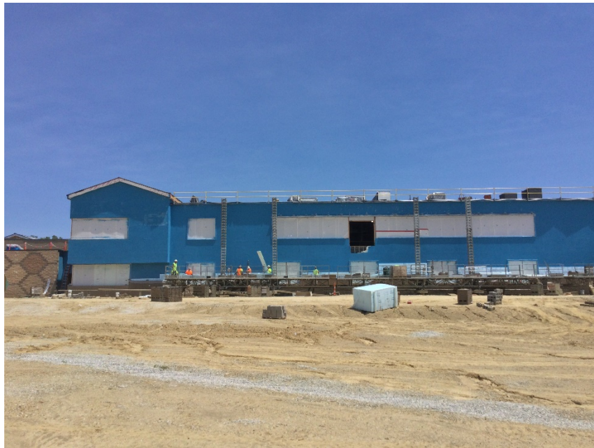
Air barrier complete and masonry veneer in progress on West side.
