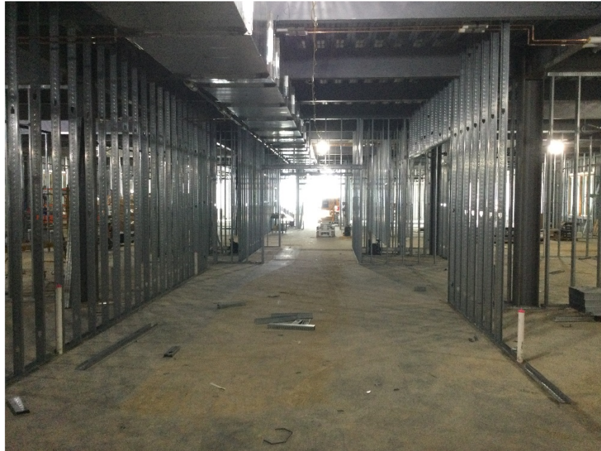
Metal studs in progress in kindergarten classroom areas.
