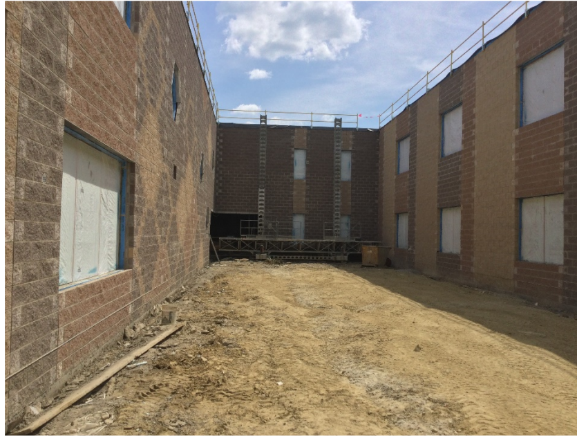
Masonry veneer complete in courtyard.
