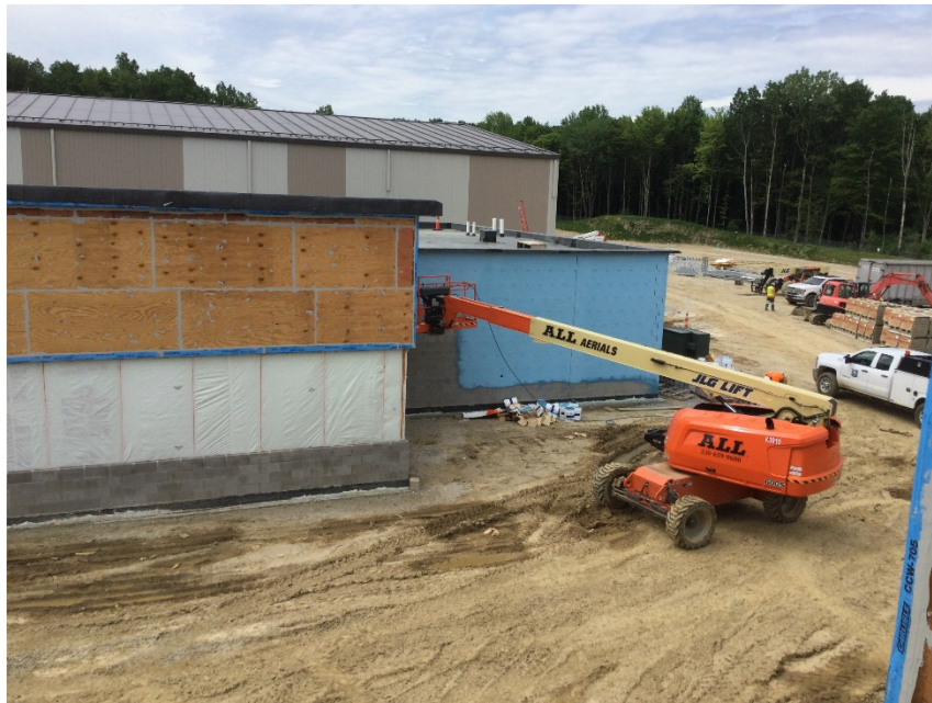
Air barrier in progress in Area 4 Dining and Mechanical areas.
