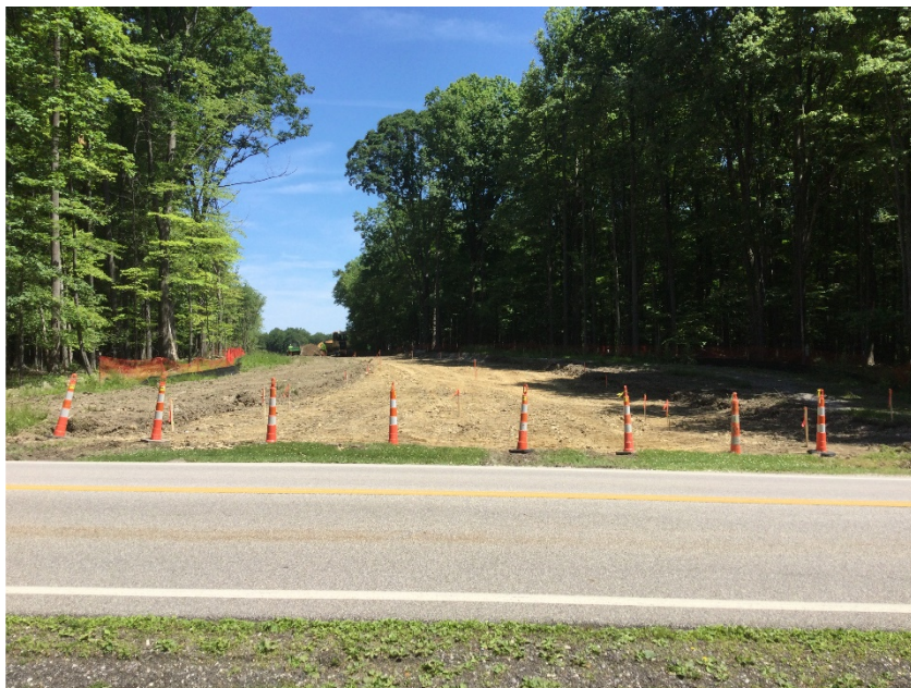
Excavation for road to Valley Parkway in progress.
