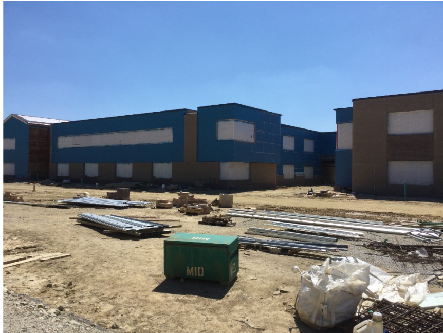
Overall view of East elevation. Air/vapor barrier and brick veneer in progress.
