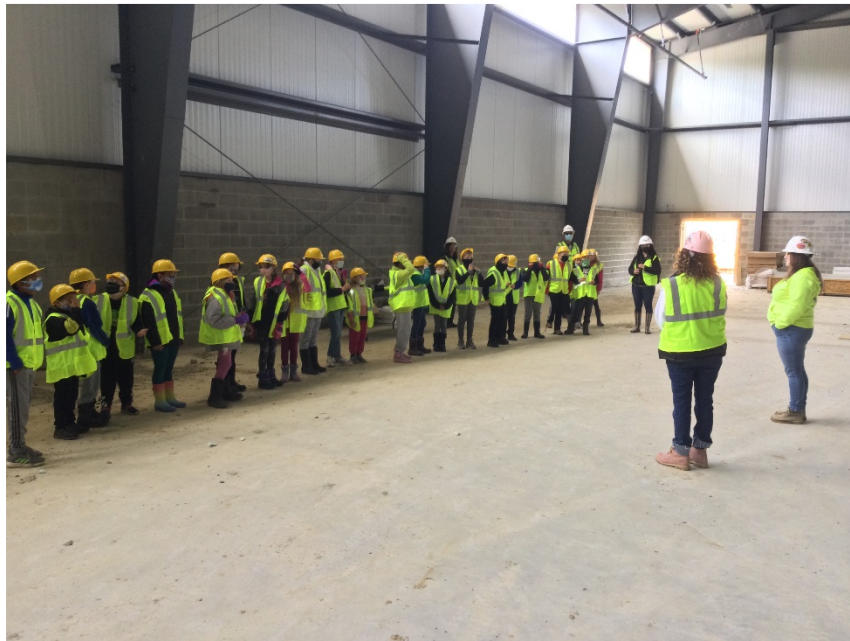
3 rd Grade student tours of the building under construction.
