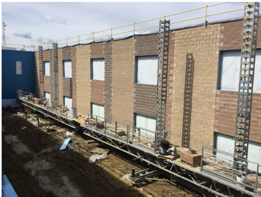
Split faced veneer complete in the Courtyard.
