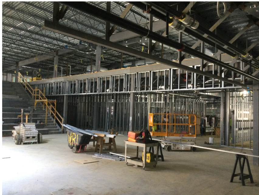
Metal wall studs in progress in Area 4.
