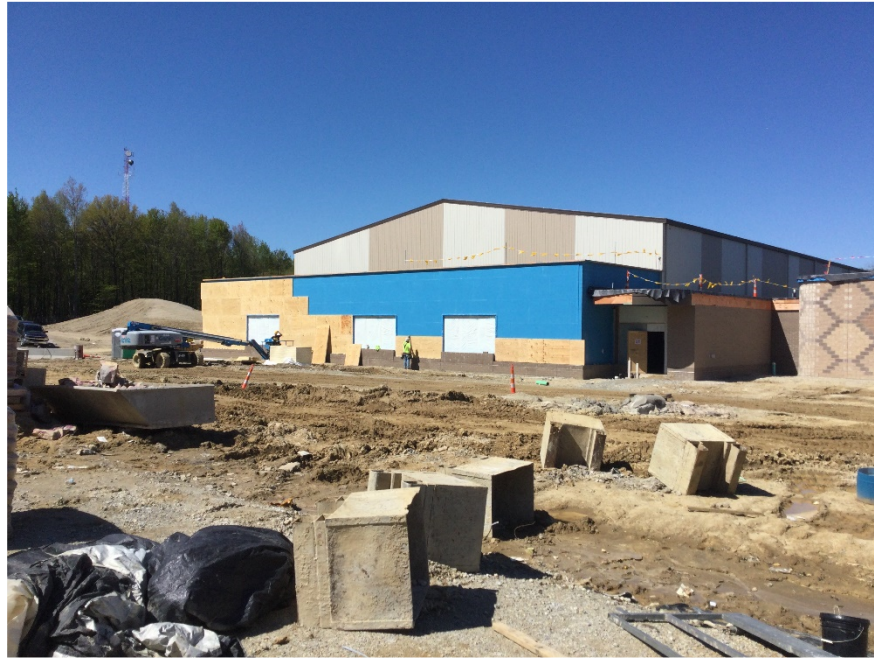
Hunter panel install in progress on Blossom Hill Field House.
