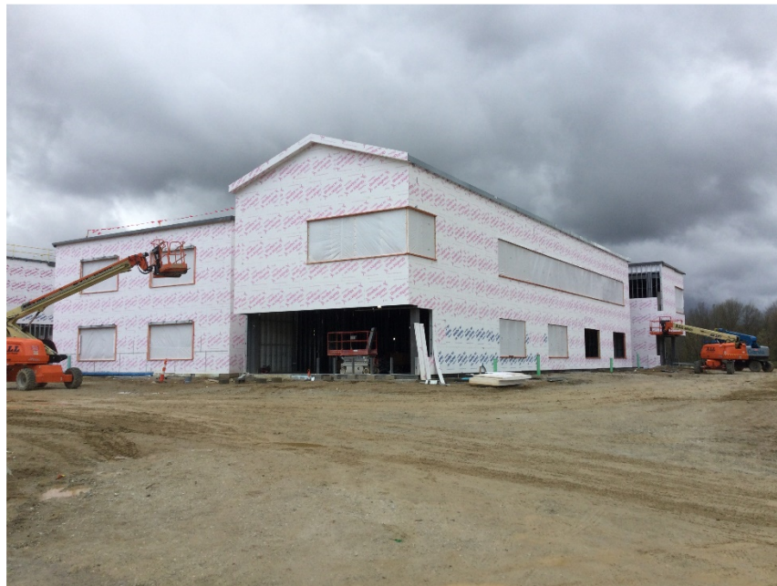
View of 4 th and 5 th grade wing exterior sheathing and enclosure in progress.
