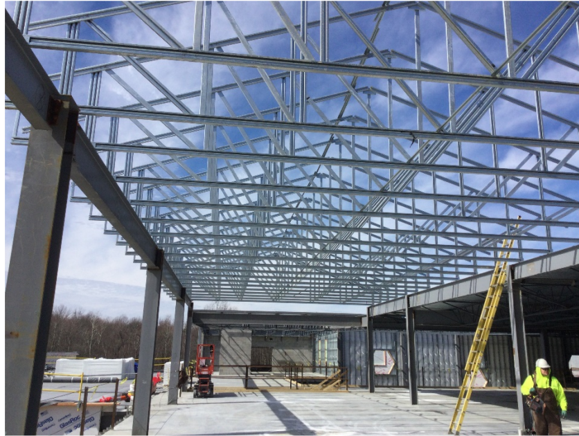
Gable roof over 2 nd and 3 rd grade wing.
