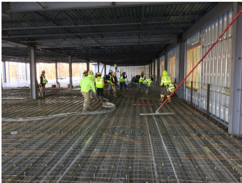
Pouring 2 nd floor concrete slab on metal deck.
