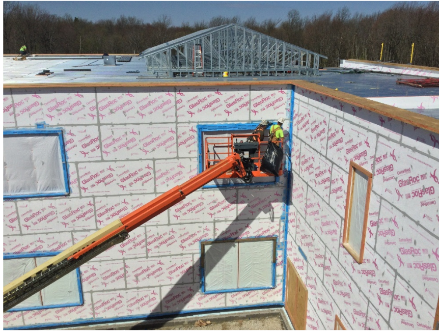
Installation of air/vapor barrier in Courtyard.
