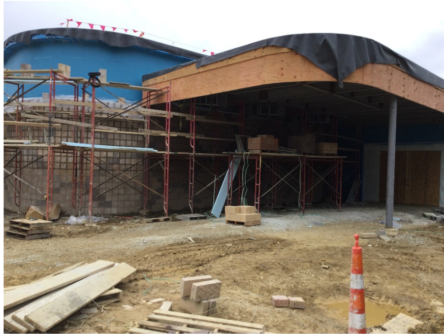
Main entrance brick veneer in progress.
