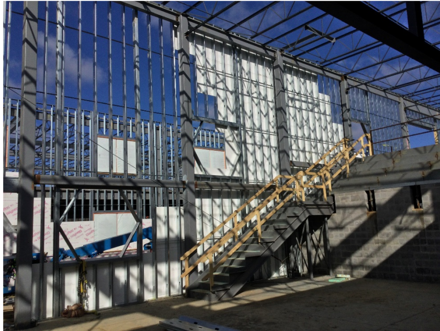
View of learning stair in progress.
