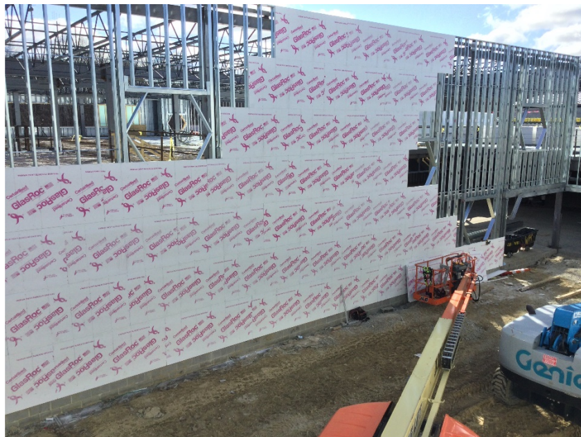
Exterior sheathing installation in progress on Courtyard walls.
