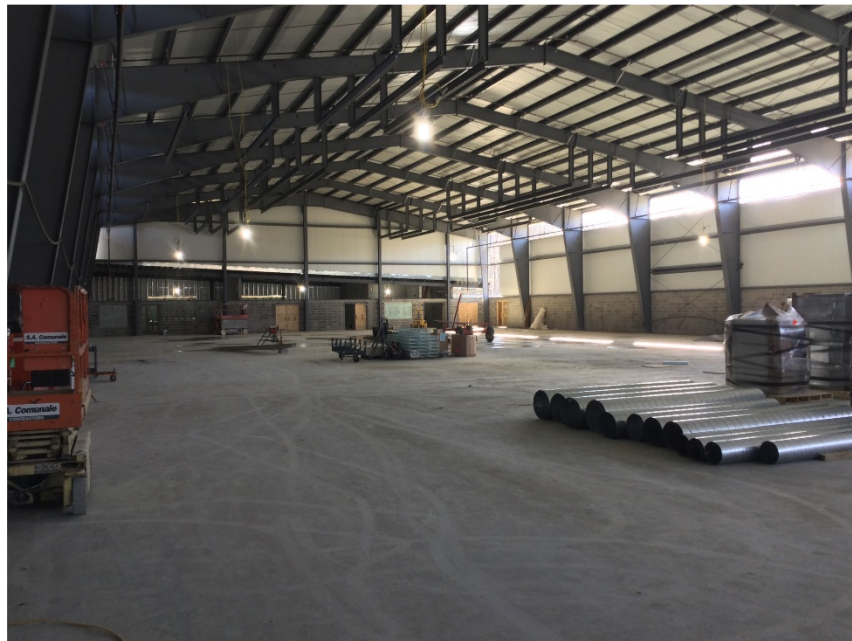
Field House metal panel installation in progress.
