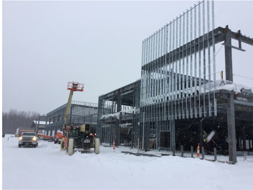
View of 4 th /5 th Grade Wing metal stud installation.
