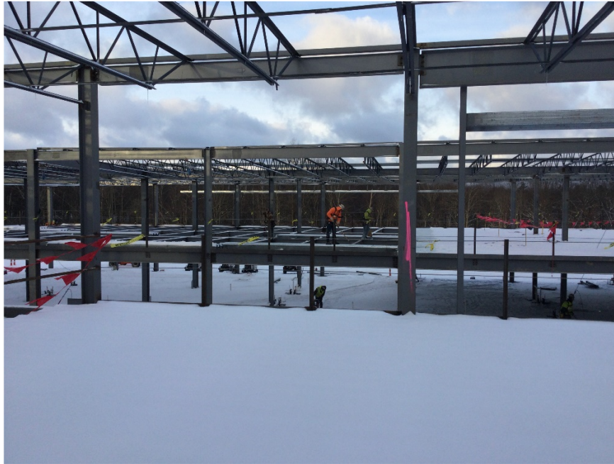
Cleaning off snow and ice off steel so 2 nd floor metal deck can be placed.
