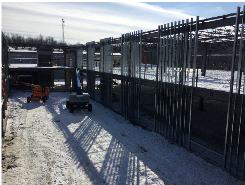
Exterior metal stud installation on Courtyard.
