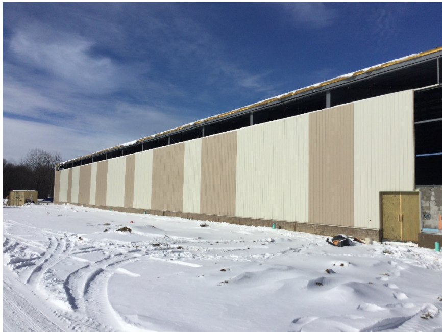
Metal panels in progress at south elevation of Field House.
