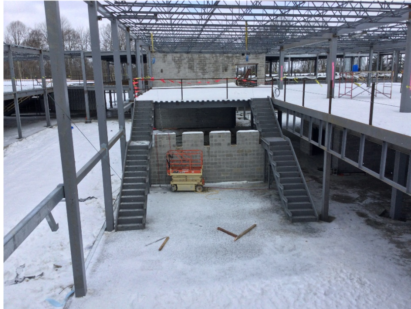
View of learning stair in progress.
