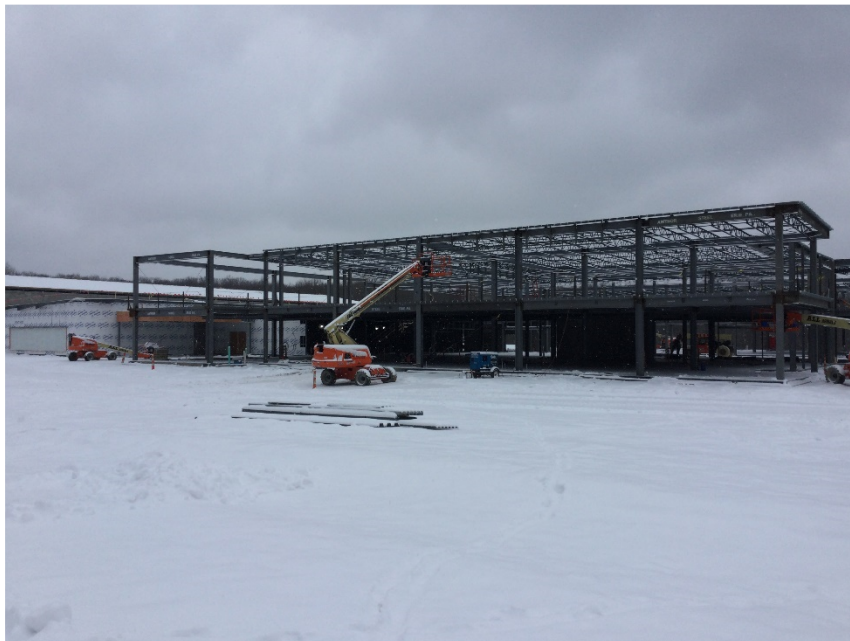
View looking at East elevation of academic wing.
