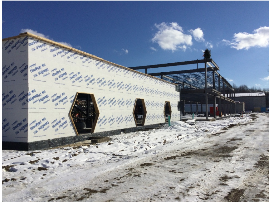
Pre-school wing with exterior sheathing complete.
