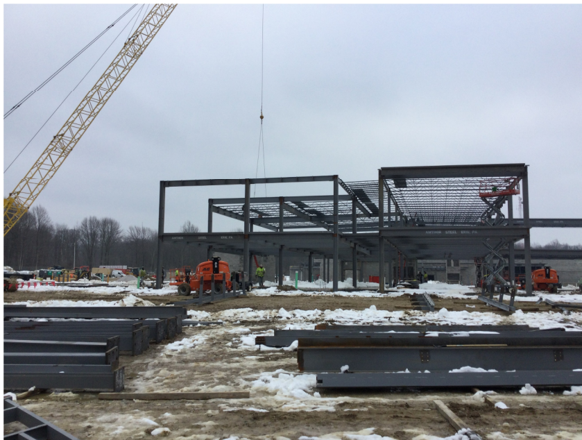
Steel erection in Area 1 (4 th /5 th Grade wing)
