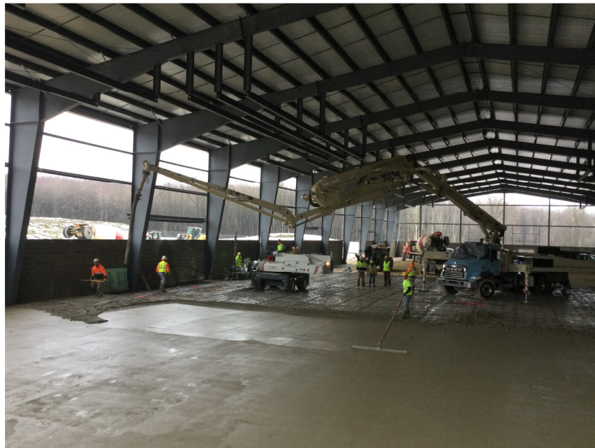
Pouring concrete slab on grade in Field House.
