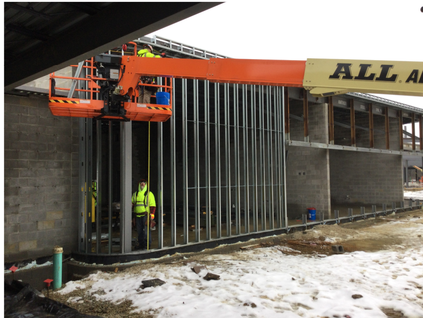
Exterior walls being framed for Band / Music rooms.
