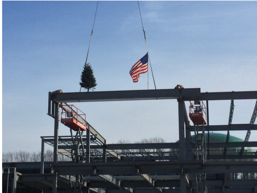
Ceremonial setting of the last piece of structural steel.
