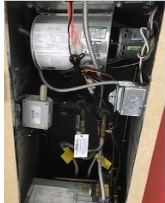
Classroom Vertical Stack Install
