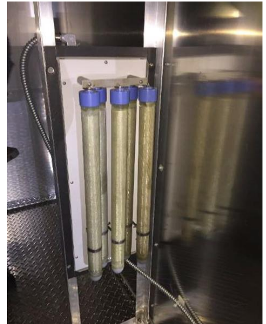
Rack or Wall Mounted in Discharge of AHU/RTU
