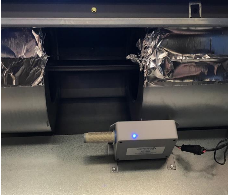
Classroom Unit Ventilator Install
