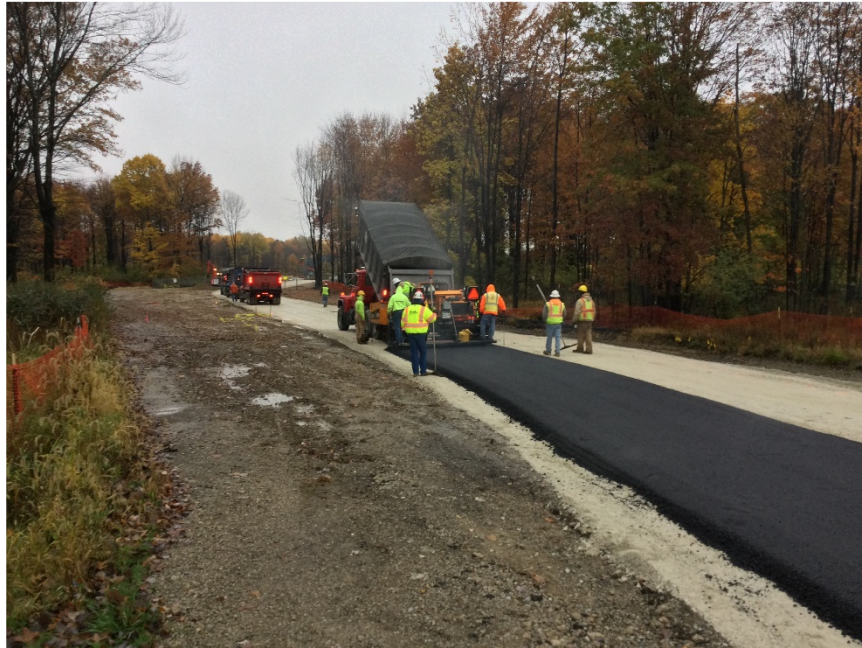
Laying base course asphalt on drive to Blossom Hill.
