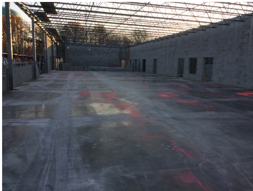
Slab on grade complete in Dining.
