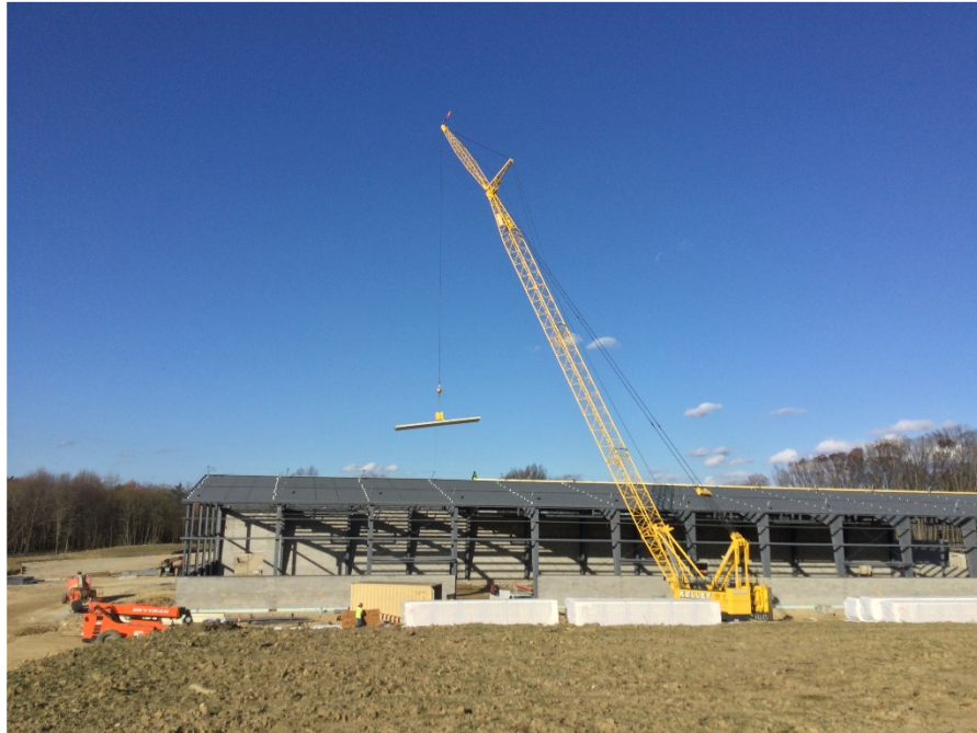
Roof panel installation in progress on Field House.
