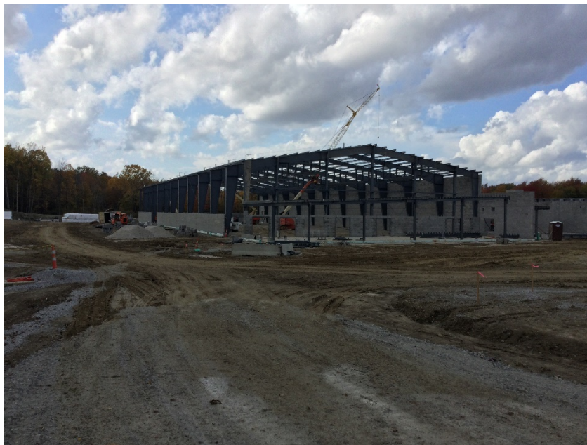
Pre-engineered metal building erection at Field House.
