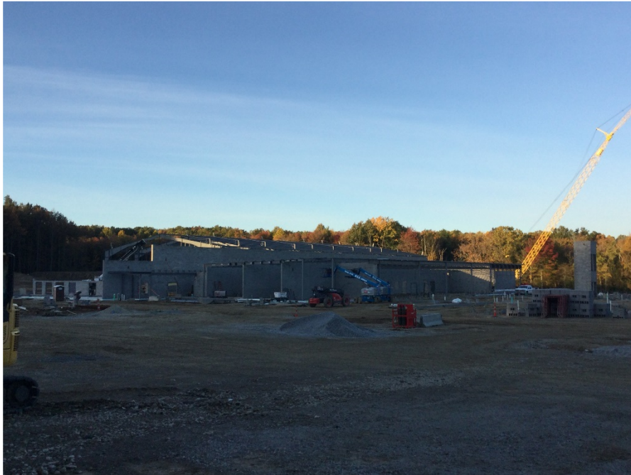
View looking southwest at Field House, Music, and Band Rooms.
