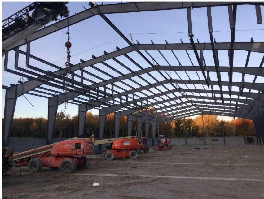
Pre-engineered metal building erection for Field House.
