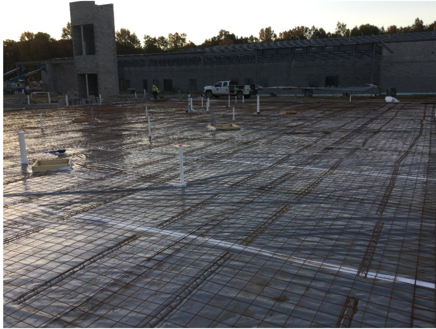
Prep for slab on grade in Area 2 classrooms.
