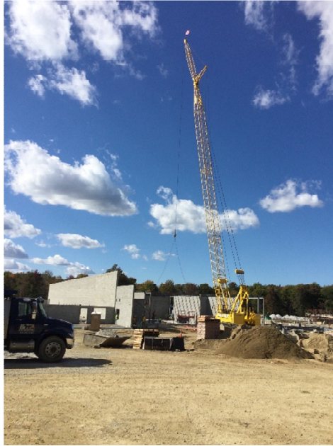
Crane for steel erection in Area 4 cafeteria and dining spaces.
