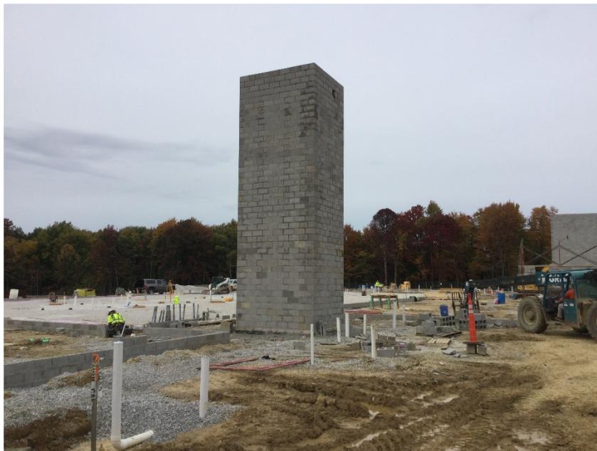
Masonry elevator shaft in Area 3 classroom.
