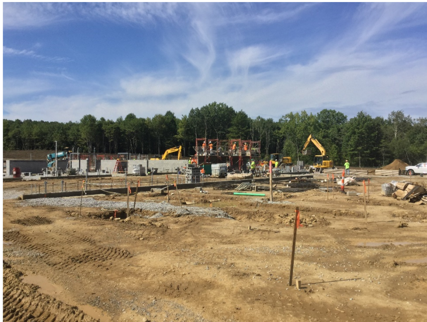
View of Student Dining masonry in progress
