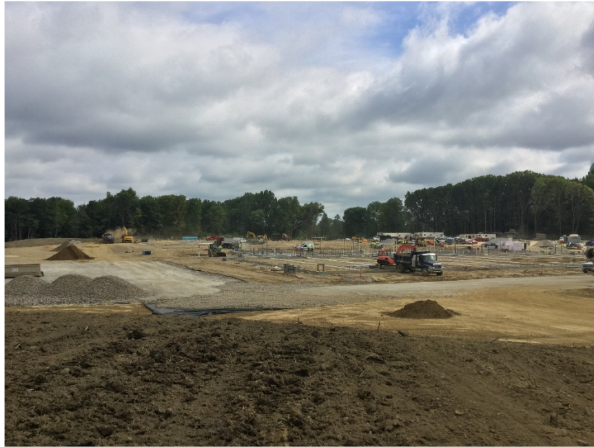
Overall view looking Northeast
