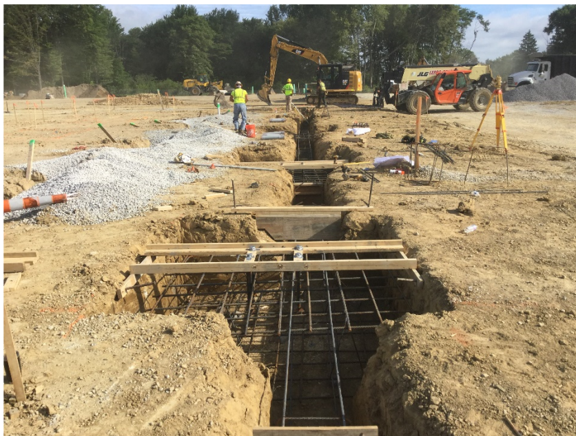
Foundation installation in Area 3
