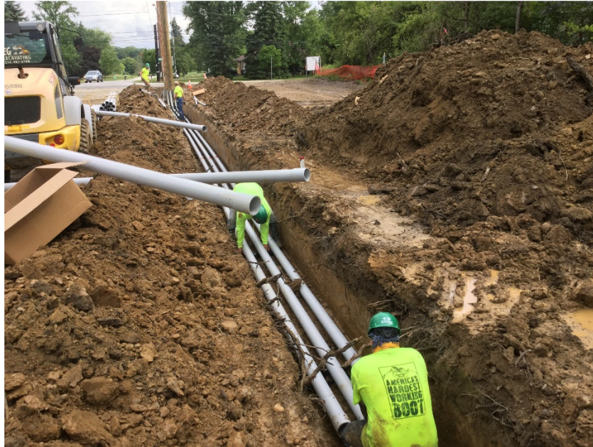
Installation of electrical and technology conduits along the entrance drive
