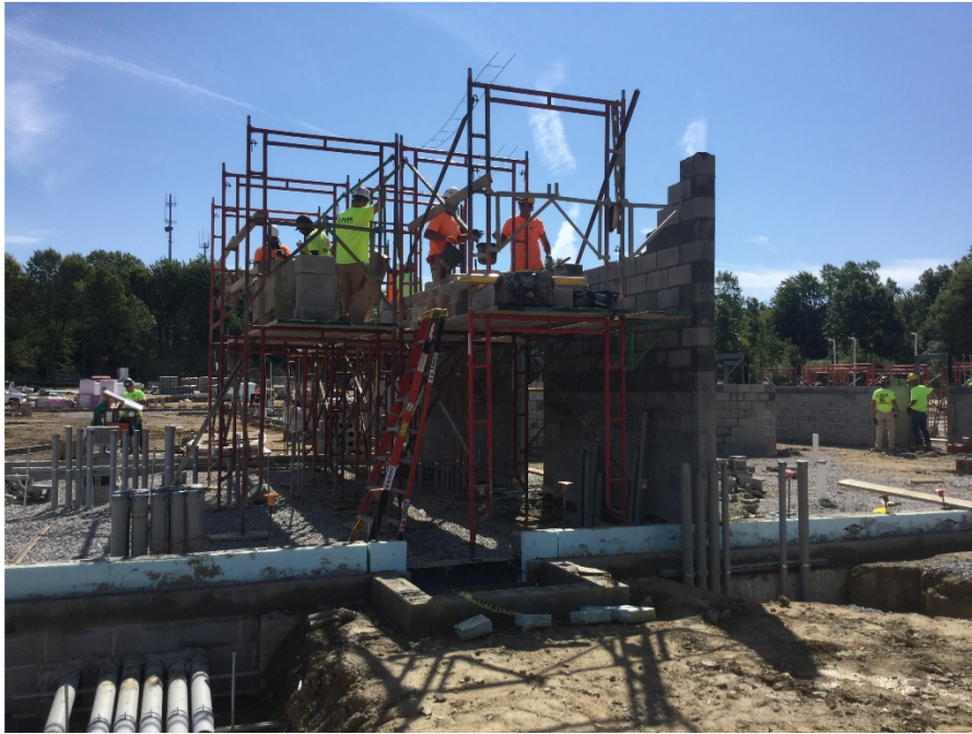
Electrical Room masonry wall installation
