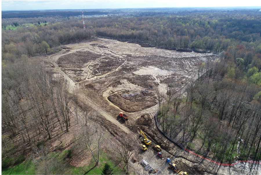
Arial view looking Southwest after trees were cleared. Topsoil removal operations have started.
