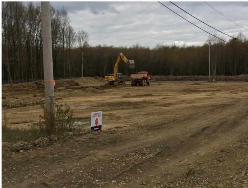
Looking Southwest. Sitework contractor continuing site cut/fill operations.
