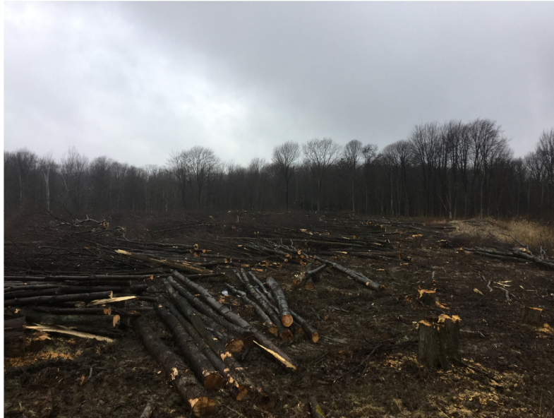
Looking Northwest showing laydown for tree clearing operations.
