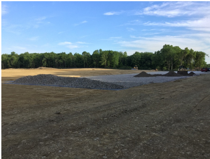
Looking North. View of stone laydown area in progress.
