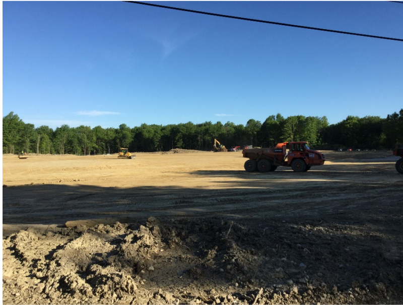
Looking Northwest at site contractor performing fill operations for the building pad.
