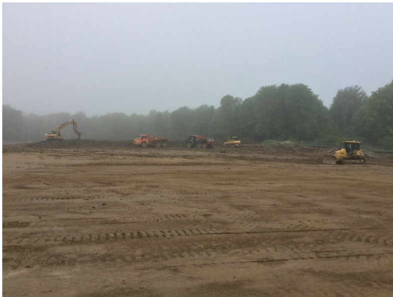
Site contractor working on filling operations and development of the building pad.
