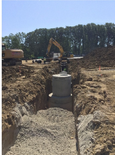
Installation for storm sewer on the north end of the site.
