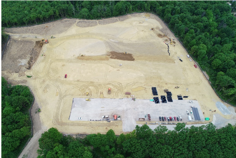
Arial view looking West showing progress on the building pad and gravel laydown area.
